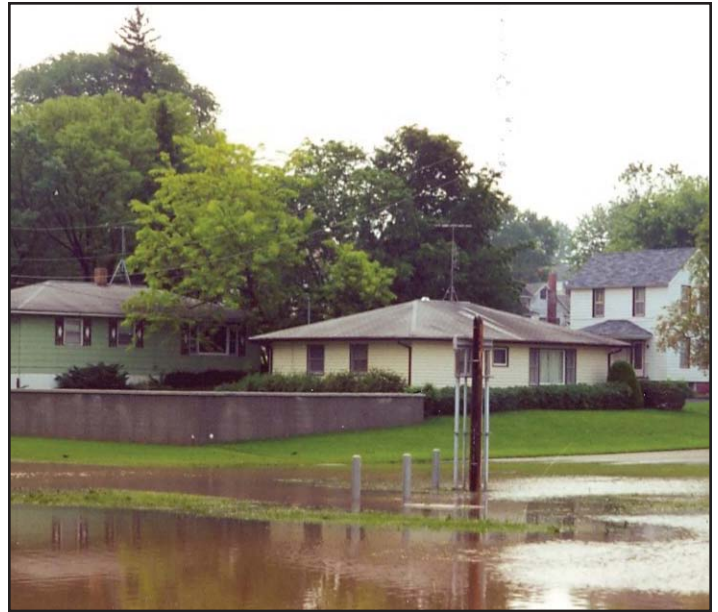
Partial barrier protects yellow house (center right). Barrier keeps high water off the property and prevents excessive erosion. Design feature prevents barrier collapse by permitting flood water to enter yard from highest end of barrier (near corner of house). Should flood waters reach this height, they would begin to fill the yard behind the wall, equalizing pressure. Removable plugs at bottom of wall permit water to drain after flood has subsided. Green house on left is elevated to protect it from floodwaters. Photo: Phil Risseeuw, Darlington
