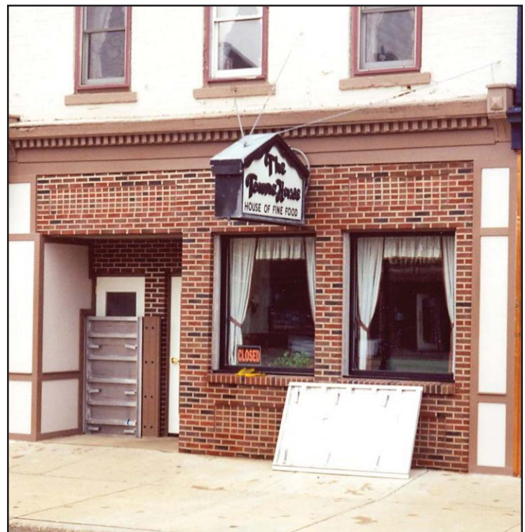
This Main Street restaurant was mitigated with hardened concrete vestibule and flood shields inside. The entrance to the apartment above the business is shielded from the outside.
