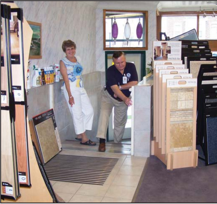
Former Darlington Mayor Bev Anderson and FEMA Mitigation Specialist Chuck Black inspect stanchions and drain cover at top of steps leading into a Main Street business. It is at this point that flood shields are attached when flooding is imminent.
