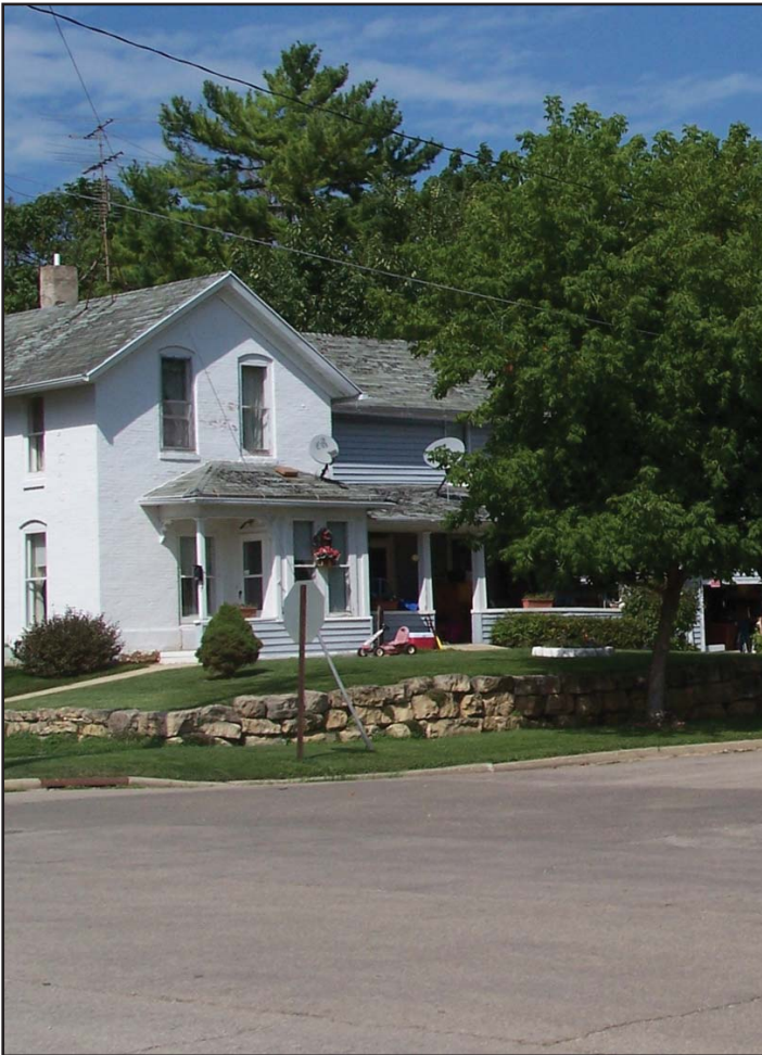
House at the end of a block of several elevated homes across street from Darlington's new ball fields. Lots and homes all are raised above the Base Flood Elevation for this neighborhood and were not flooded during the June 2008 flood.
