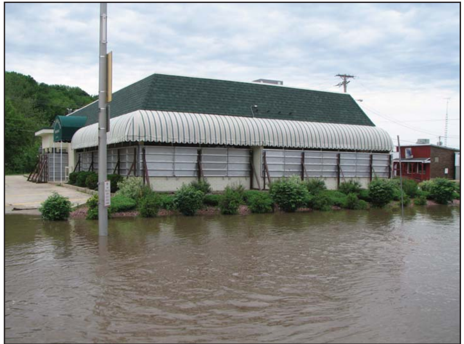
A Darlington business with flood shields installed shown during a 1998 flood.
